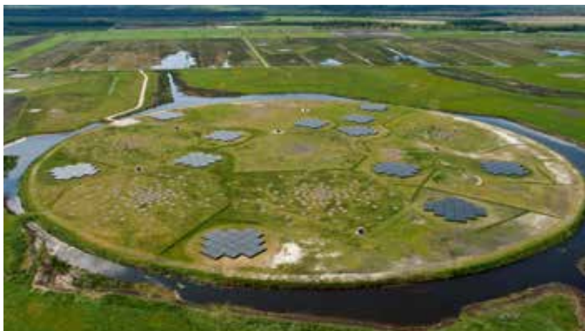
The LOFAR superterp houses six antenna stations and is part of the gigantic collection of antennas that span half of Europe. Due to its size LOFAR is able to scan frequencies that are not accessible to most other telescopes.
